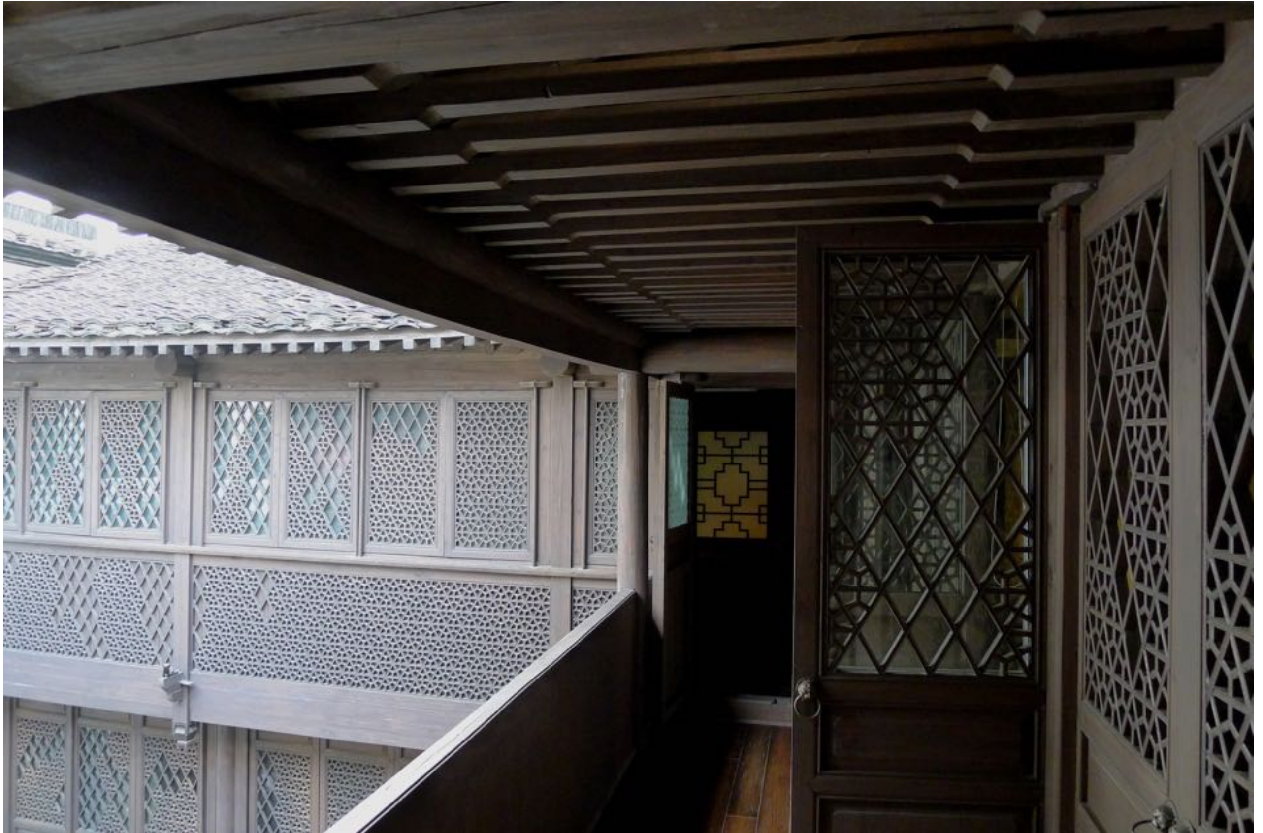
Shaoxing Guesthouse Renovation eines traditionellen Hofhauses
