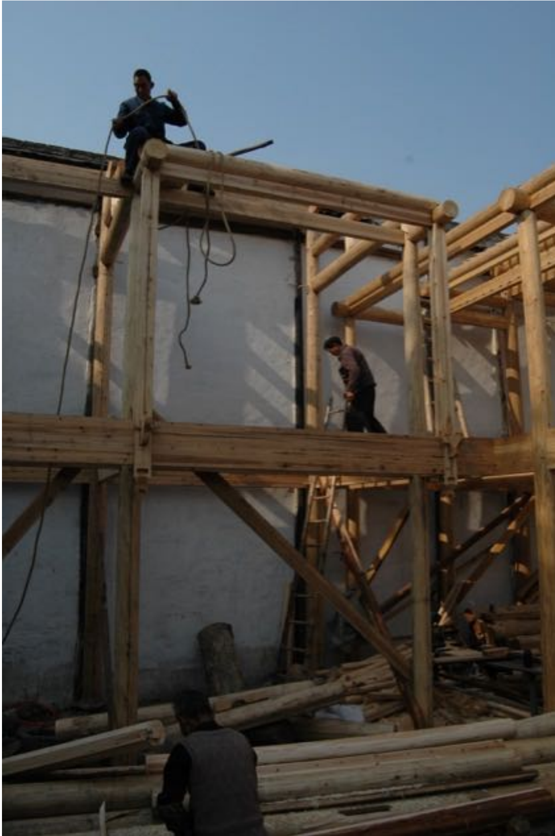
Shaoxing Guesthouse Renovation eines traditionellen Hofhauses
