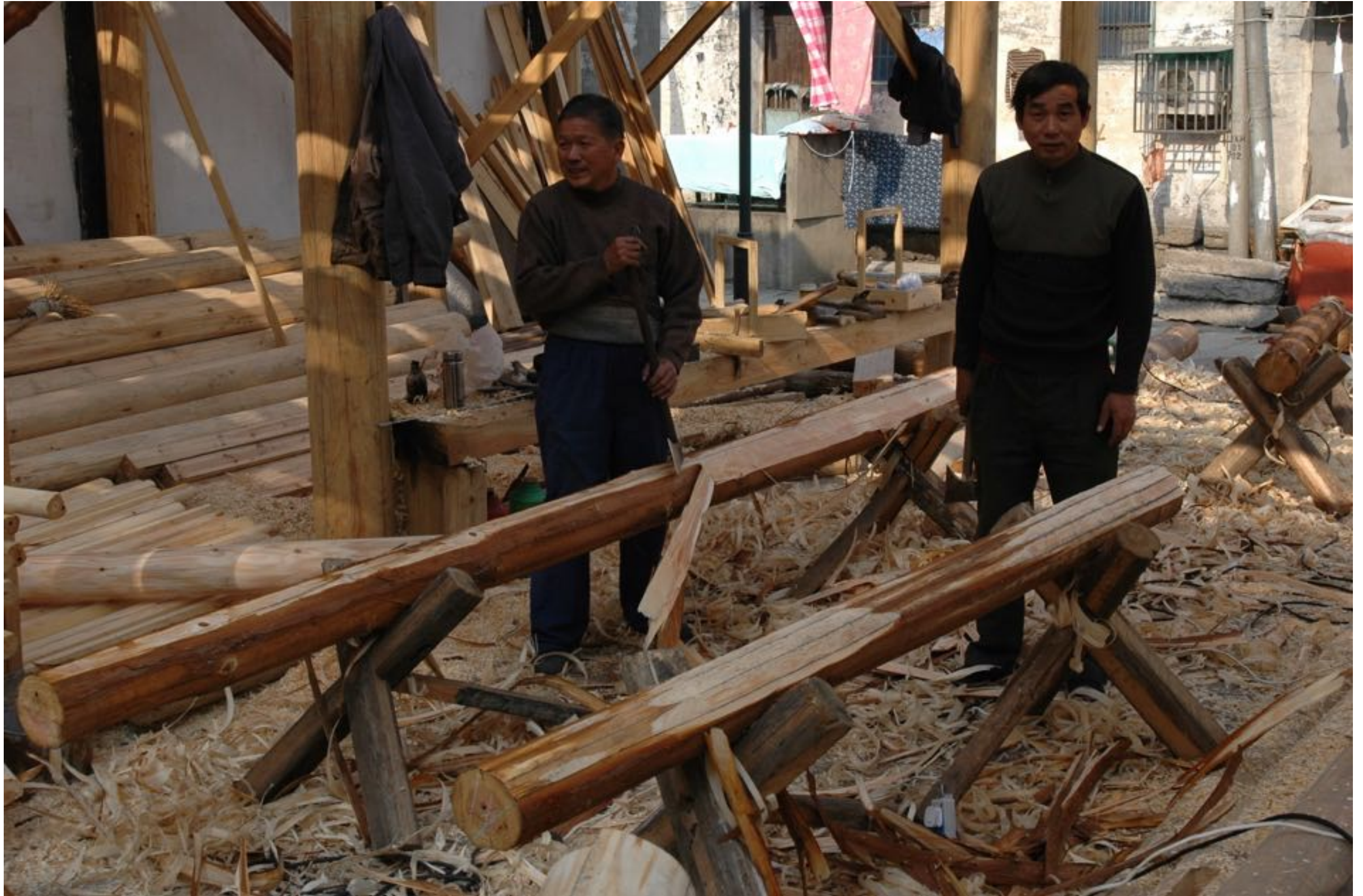
Shaoxing Guesthouse Renovation eines traditionellen Hofhauses
